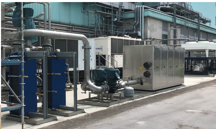
Figure 3: Heatpump “High temperature Heat Pump for heat recovery”.
