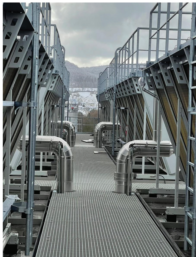
Figure 5: Drycoolers “Drycoolers to provide freecooling up to 14°C Outside temperature”.
