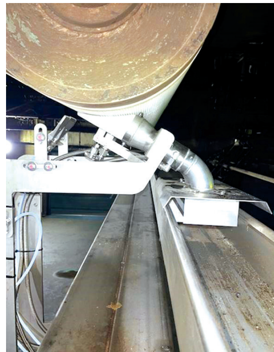
Figure 2: Power Cleaner 2.0 on Bottom Fabric.
