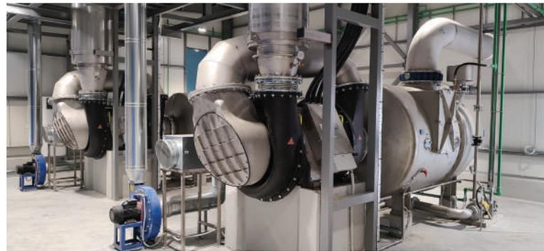
**Figure 1: RunEco EP Turbo Blowers are modern blowers with integrated high-speed motor controlled by a frequency converter: rotation speed and vacuum level can be adjusted according to the process requirements.**
