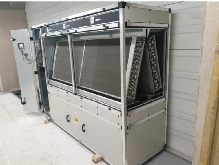
**Figure 2: The Climate Cabinet: “Special Engineered Climate cabinet for the paper industry, with Siemens S7 control unit and A-shape coil to enable high natural cooling share for a year”.**
