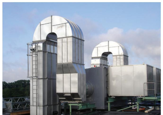
*Figure 6: Heat recovery, as an important part of the RunEco solution, cuts down papermaking energy costs radically because the system reuses heat to replace primary energy sources.*
