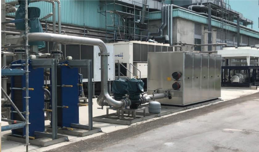
**Figure 3: Heatpump “High temperature Heat Pump for heat recovery”.**
