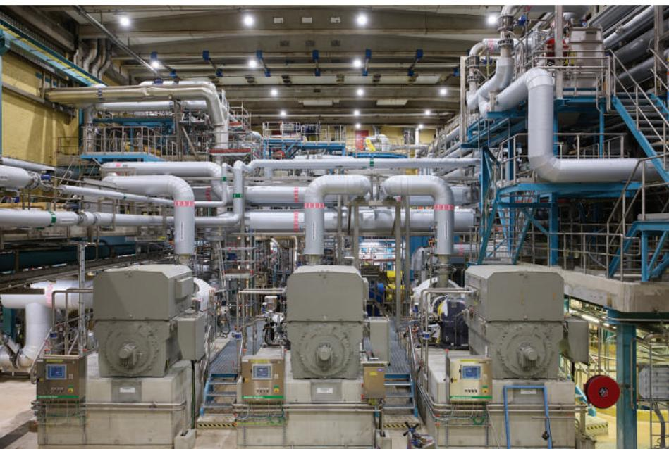
**Figure 7: The three low consistency refiners.**
